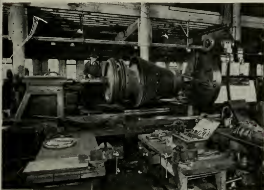
At top, left: Checking rotor from Low Pressure turbine for trueness prior to removing blades. Right: Reblading lower half of LP casing.
